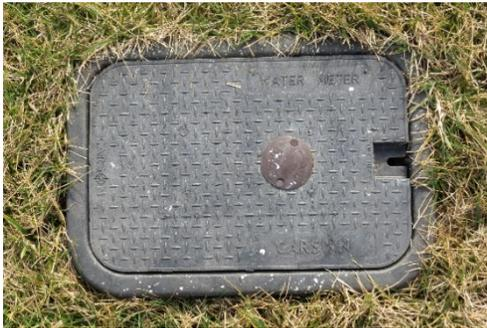
Figure 1. Typical Water Meter Housing Cover
