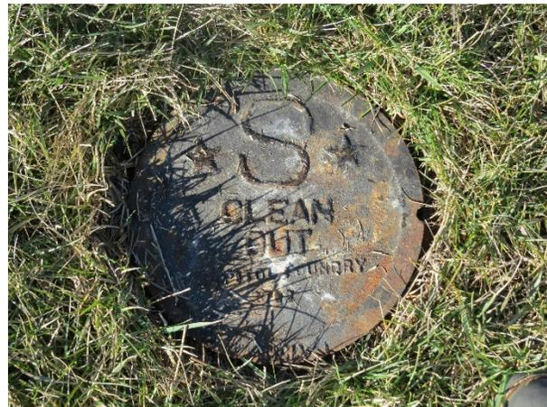
Figure 2. Typical KGCSA Sewer Cleanout
