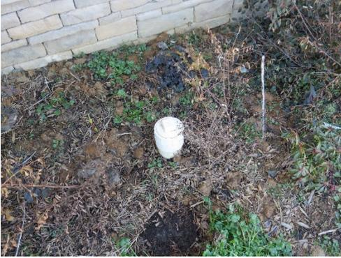
*Figure 3. Typical Residential Sewer Cleanout*
