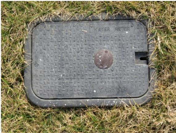
Figure 1. Typical KGCSA Water Meter Housing
